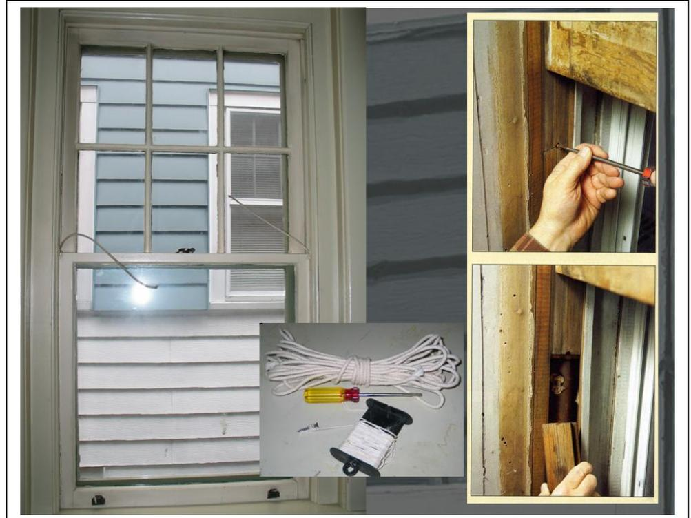
Do not cut the final length of the new cord until it is tied to the weight and the weight is back in the cavity. The length is determined by lifting the weight to the top and aligning the end with the knot hole in the sash when the sash is in the lower-most position. This assures that there is not too much slack in the rope and that the window is sufficiently suspended and counterweighted with the weight.
