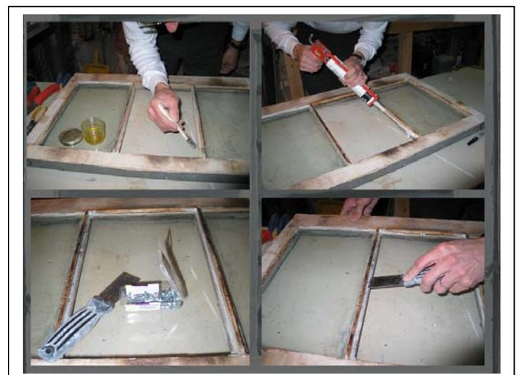
With the glass pane out, the remaining putty can be removed from the wood by scraping or sanding. Putty that remains stuck to the pane of glass can be removed by adding sufficient linseed oil to soften the hard putty.
