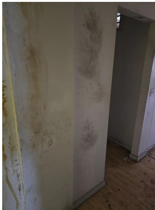
Mold and water damage on Entry Hall D Wall
