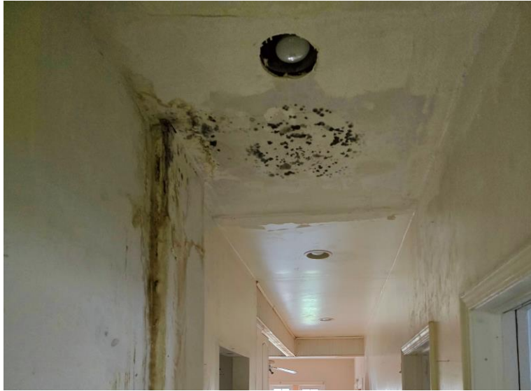
Mold on Entry Hall ceiling
